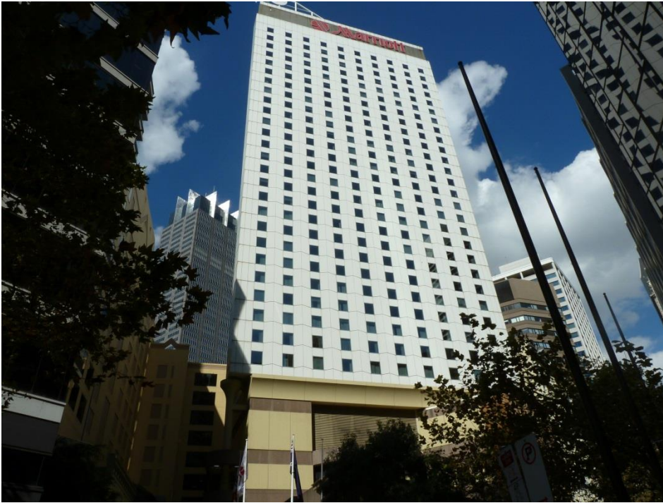
Figure 15: View of adjacent Marriot Hotel fronting Pitt Street to the east
