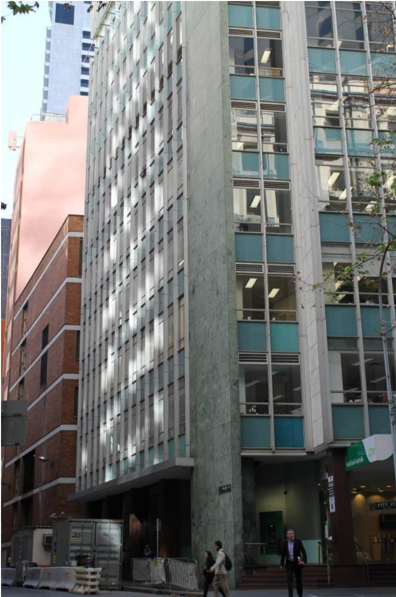
Figure 12: Dalley Street elevation of existing buildings (view west)
