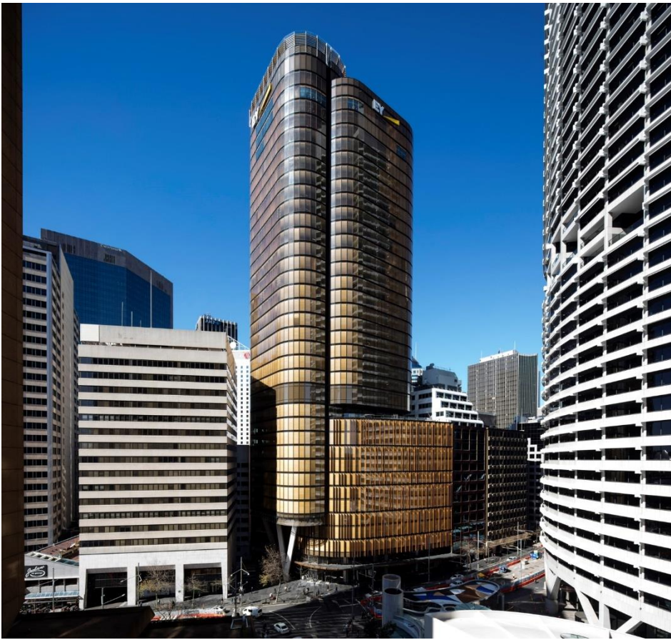
Figure 17: View of 200 George Street (centre) - 2017
