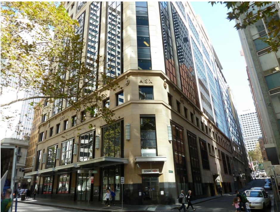
Figure 16: ASX building to the south fronting Dalley and Pitt Streets
