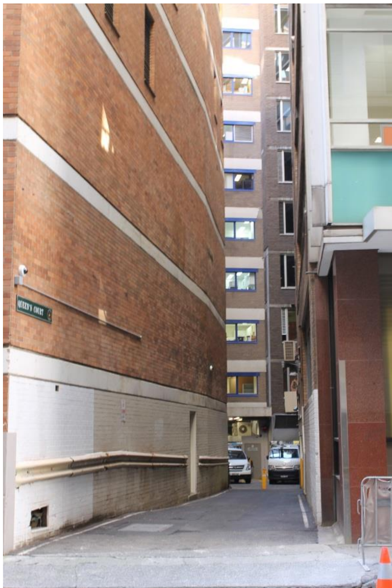
Figure 14: Queens Court elevation of existing buildings (looking north)
