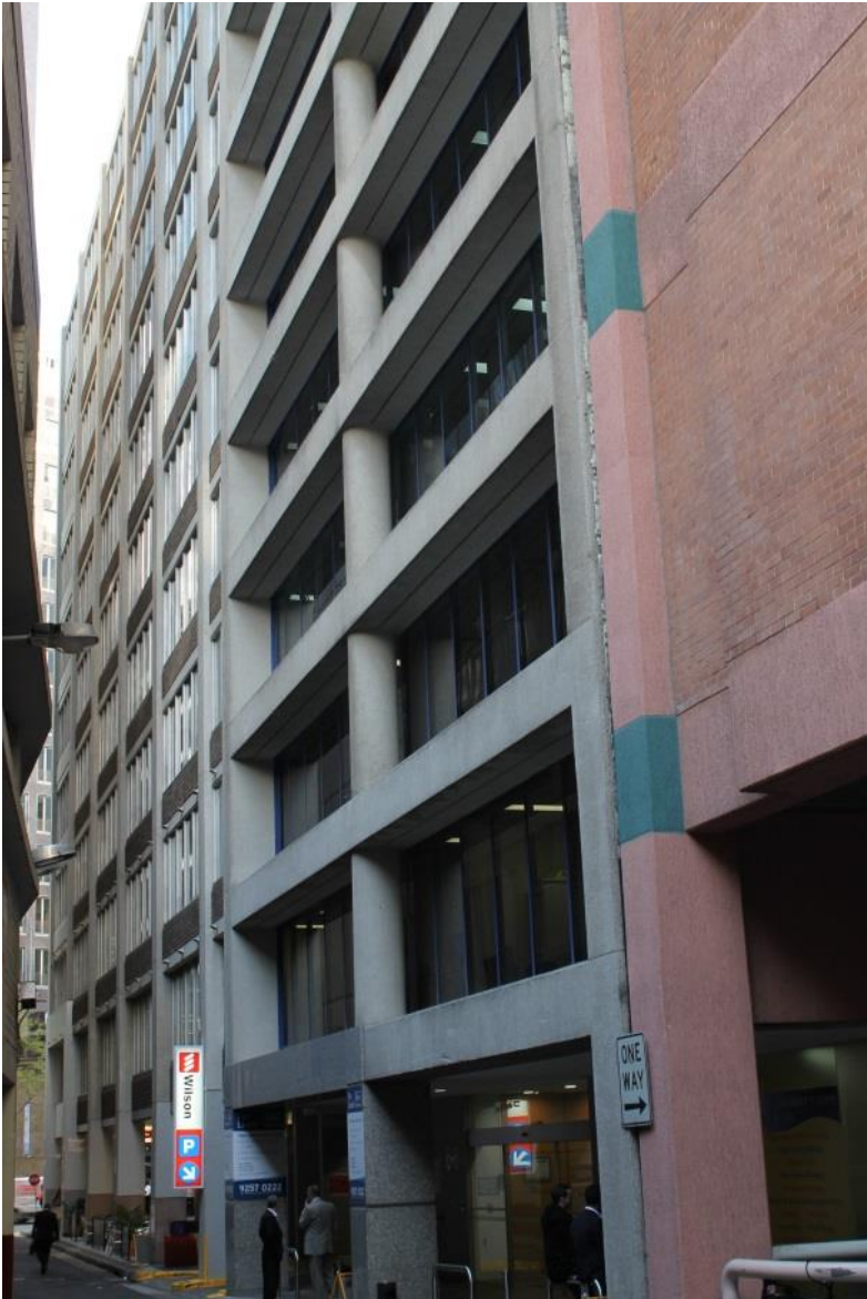
Figure 11: Underwood Street elevation of existing buildings (view east)
